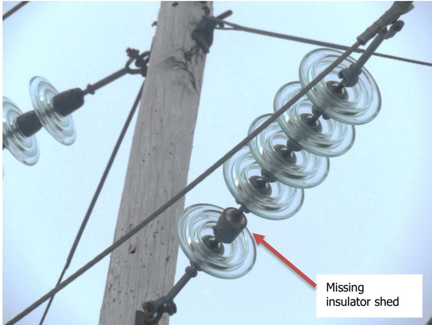
Figure B-7: Broken Insulator Shed
