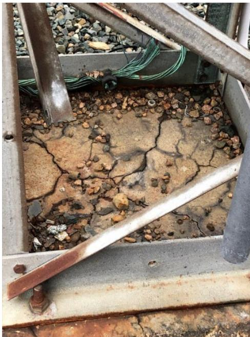
*Figure B-5: Deteriorated 12.5 kV Concrete Pier Foundation*
