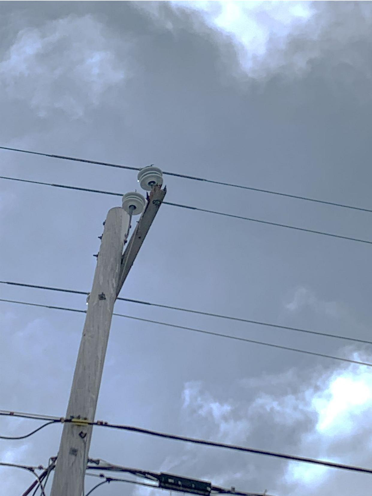
Figure C-2: Deteriorated Crossarm and Porcelain 2-Piece Insulators
