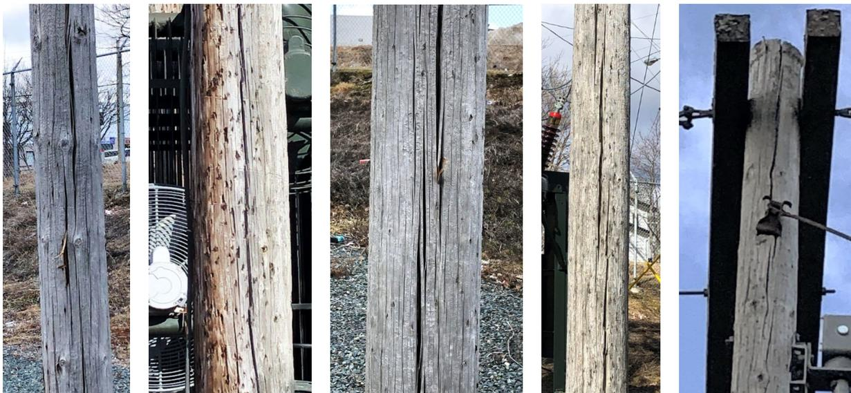
*Figure B-3: Deteriorated Wood Poles*
