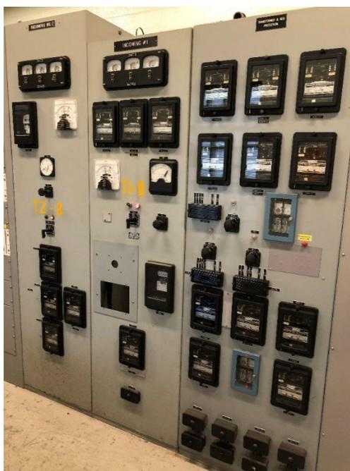
Figure B-6: MOL-T1 and MOL-T2 Protection Equipment
