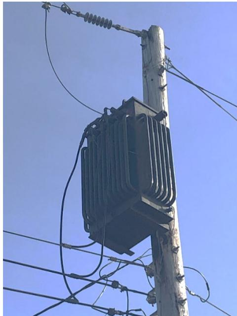
*Figure 4: Deteriorated Pole and Vintage Transformer*
