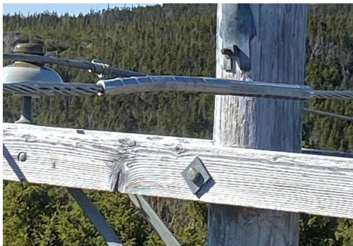
*Figure 4: 2/0 ACSR Conductor Repair*
