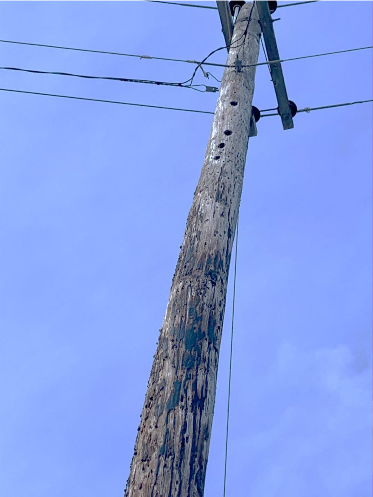
Figure C-4: Deteriorated Pole with Woodpecker Holes
