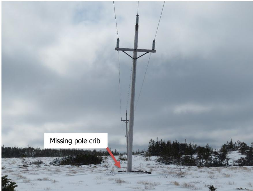
Figure B-8: Pole Crib Deteriorated/Pole Leaning
