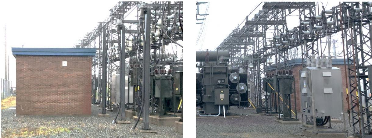
*Figure B-8: MOL Substation Control Building with Insufficient Clearances to 12.5 kV Structure*
