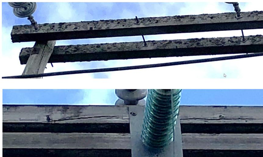
Figure B-4: Deteriorated Wood Crossarms
