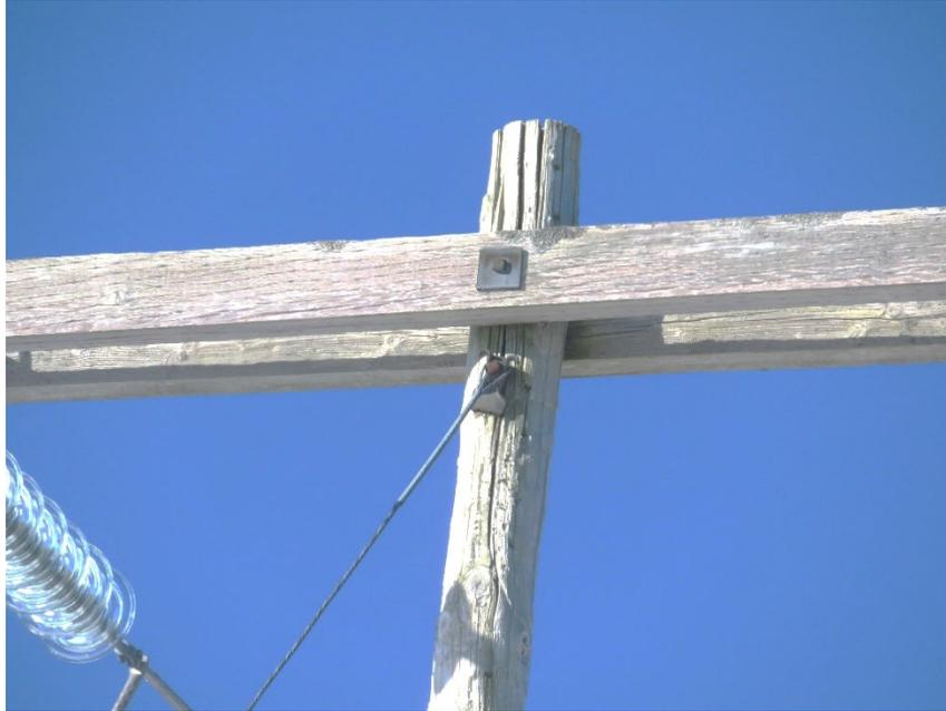
Figure B-11: Deteriorated Pole Top
