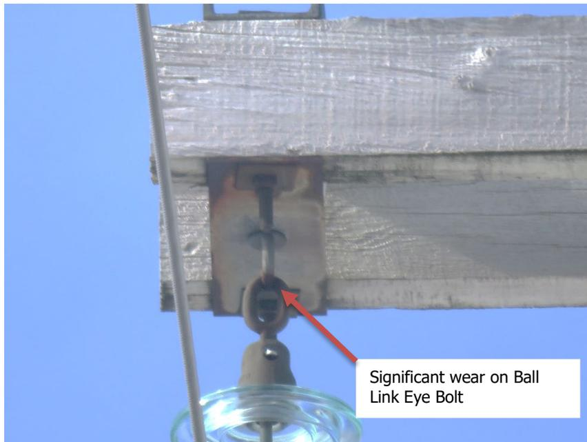
Figure B-12: Worn Ball Link Eye Bolt
