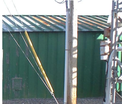
Figure A-8: WAL Substation Building Roof Showing Signs of Deterioration
