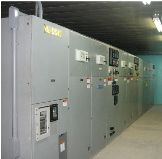
*Figure A-2: WAL Substation 12.5 kV Switchgear Front Layout and Protection and Controls*
