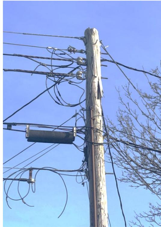
*Figure 3: Deteriorated Secondary Pole*
