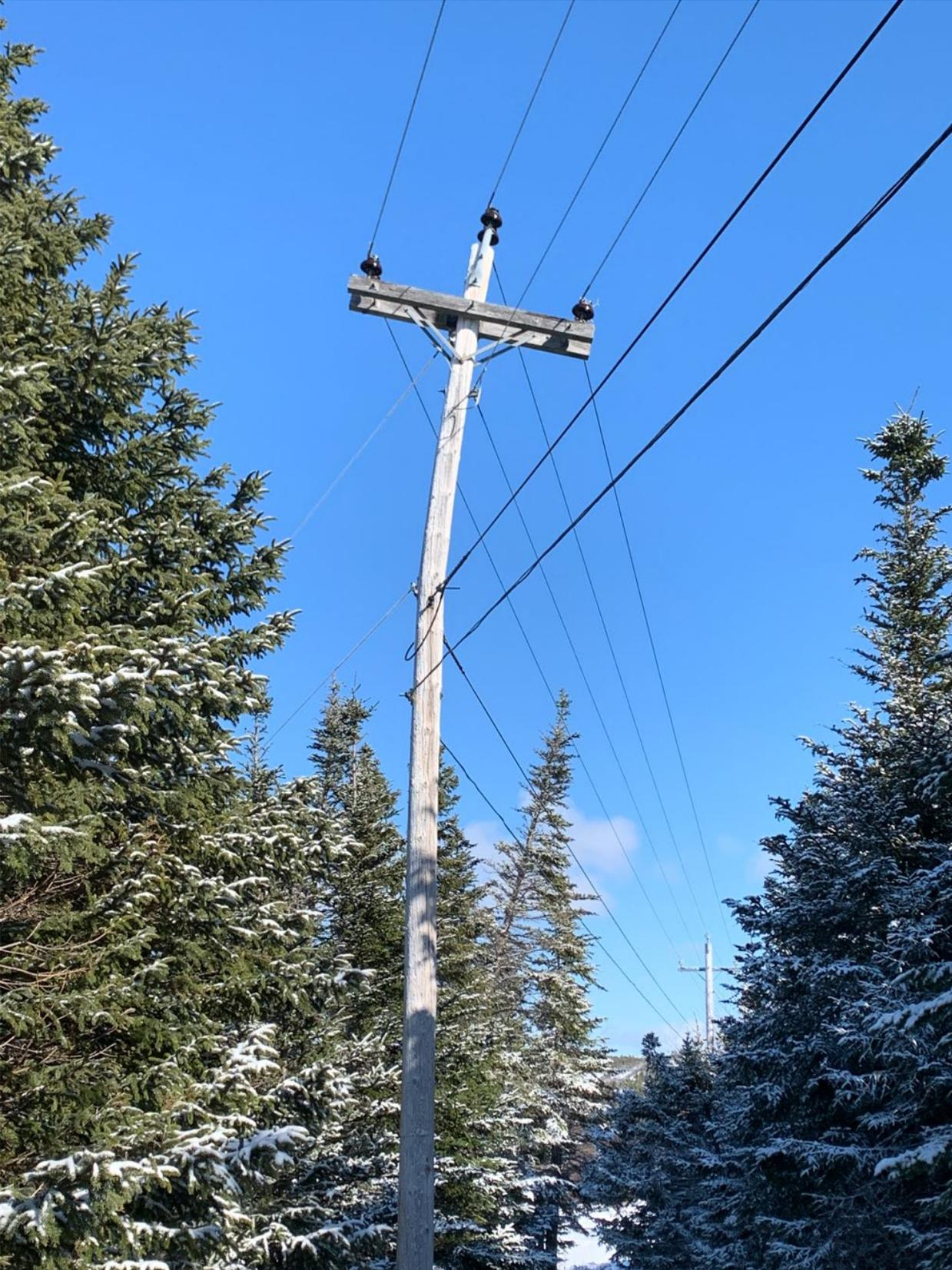
Figure C-5: Bent Pole and Vintage Insulators
